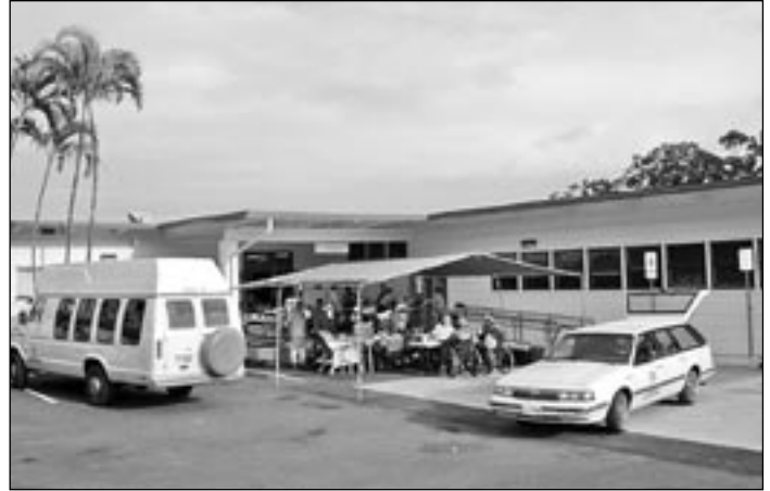
Parking Lot area converted to a Dining Room and Recreation area.
